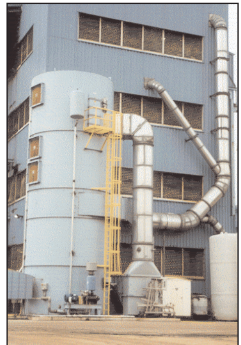
This is an Air Cure bolt together 676RF10 handling coal dust at a coal crusher house.
