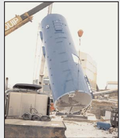
The all-welded design enables the filter to be lifted in one piece including the skirt support.
